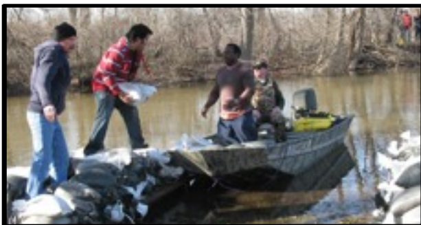
Volunteers work to shore up the levy at Center Lake in Warsaw Indiana
